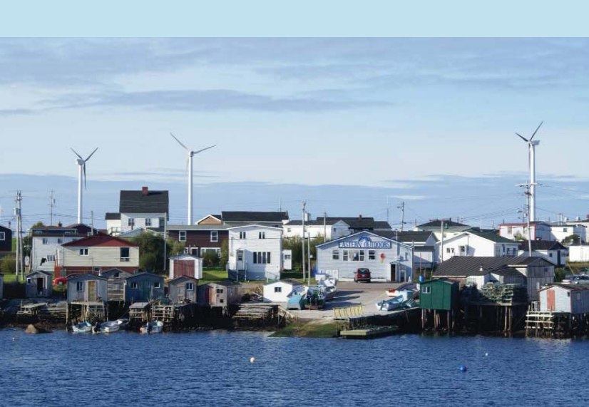
Wind turbines in Ramea, NL Image Source: Nalcor Energy
