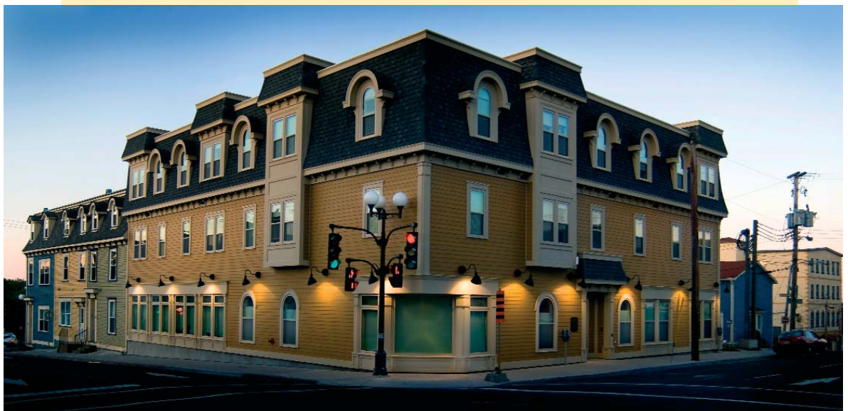
Stella Burry Building, St. John's, NL Image Source: Greg Locke photo, courtesy of Stella Burry Community Service
