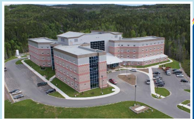
Corner Brook Long-Term Care Facility, NL Image Source: Department of Transportation and Works
