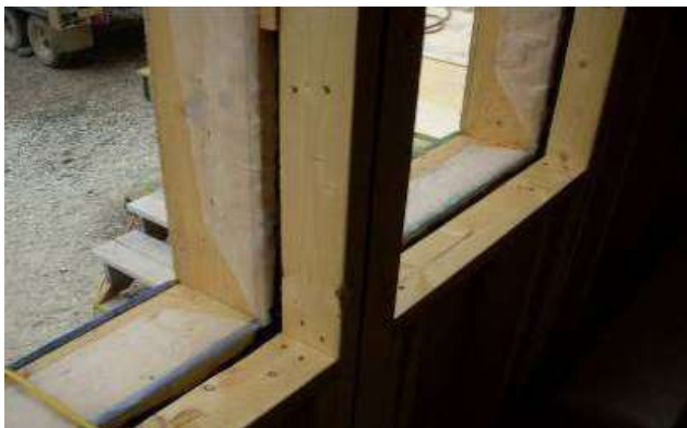
Figures 60 and 61: A double wall and solar features on the E9 House (Craig 2009)
