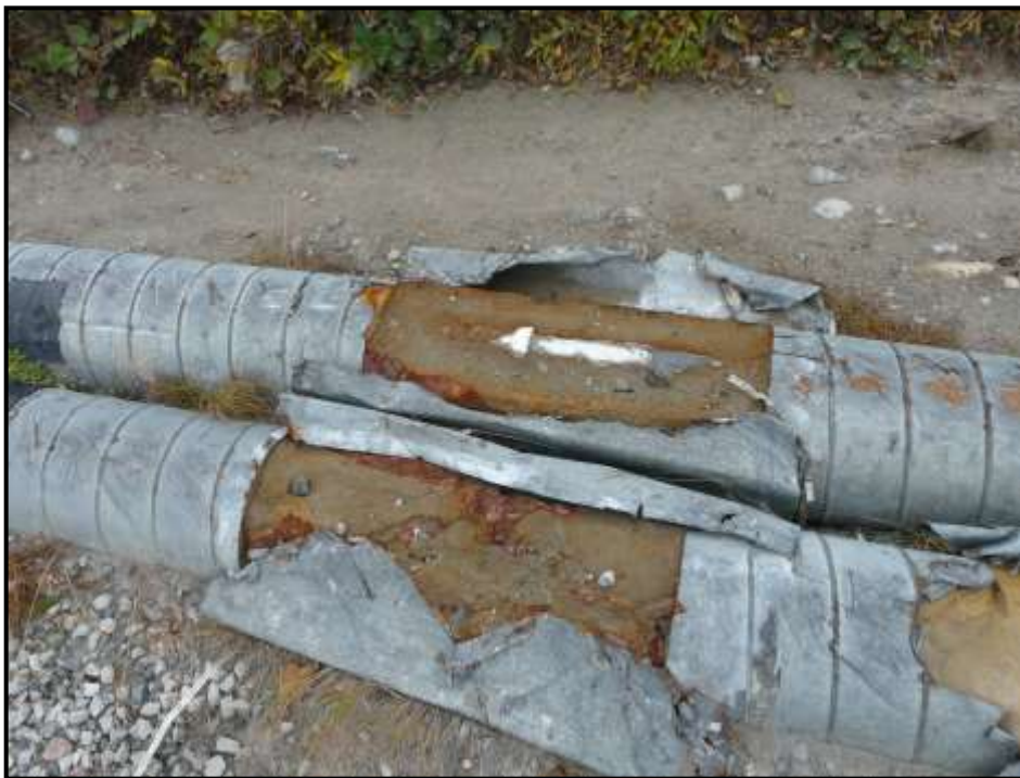
Previous water and sewer pipes
