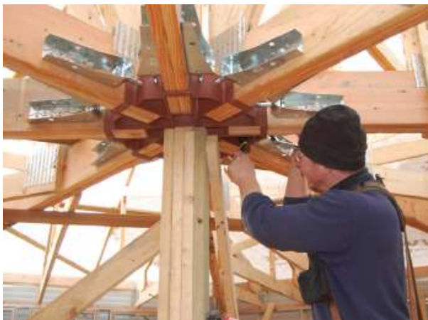
Figures 127 and 128: The roof truss tension bracket and off set wall with bracing (CCHRC 2011)
