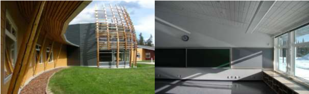
Figure 95: The importance of balancing the need for long overhangs and windows that will allow low winter light is demonstrated in the design for Tantalus School, Carmacks, Yukon by Kobayashi Zedda Architects (Zedda 2010)
