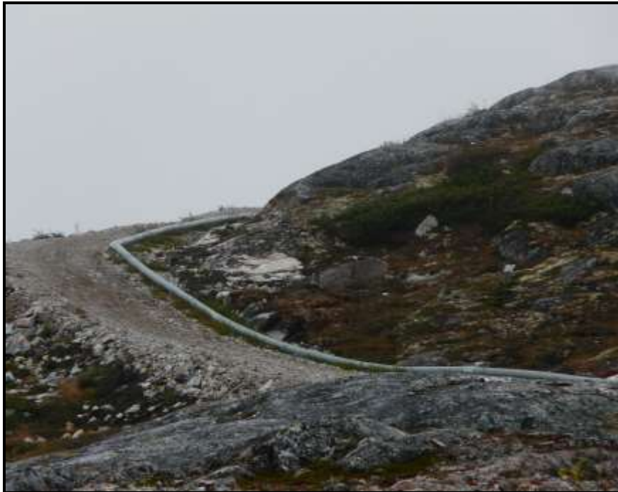
The two surface water supplies are connected by this water pipe. Gravity moves the water from the pond located at a higher elevation to the lower pond when additional water is needed.
