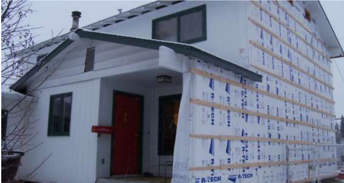
Figure 71: A REMOTE Wall Retrofit in Alaska (CCHRC 2012)
