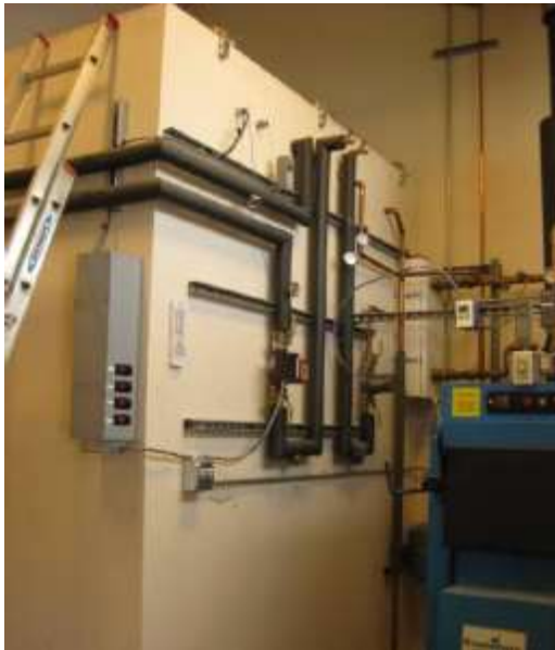
Figures 90 and 91: Thermal Storage Tank and Alaskan Windmill (Craven et al 2013)
