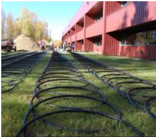
Figures 107 and 108: Ground loops for installation at Weller School and Heat pump units at the Juneau Airport. (Craven et al 2013)
