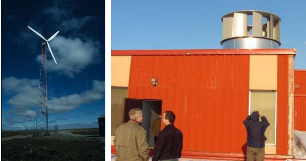
Figures 76 and 77: Windmill at Rankin Inlet, Nunavut / Vertica Vertical Wind Axis Turbine (Semple 2009)
