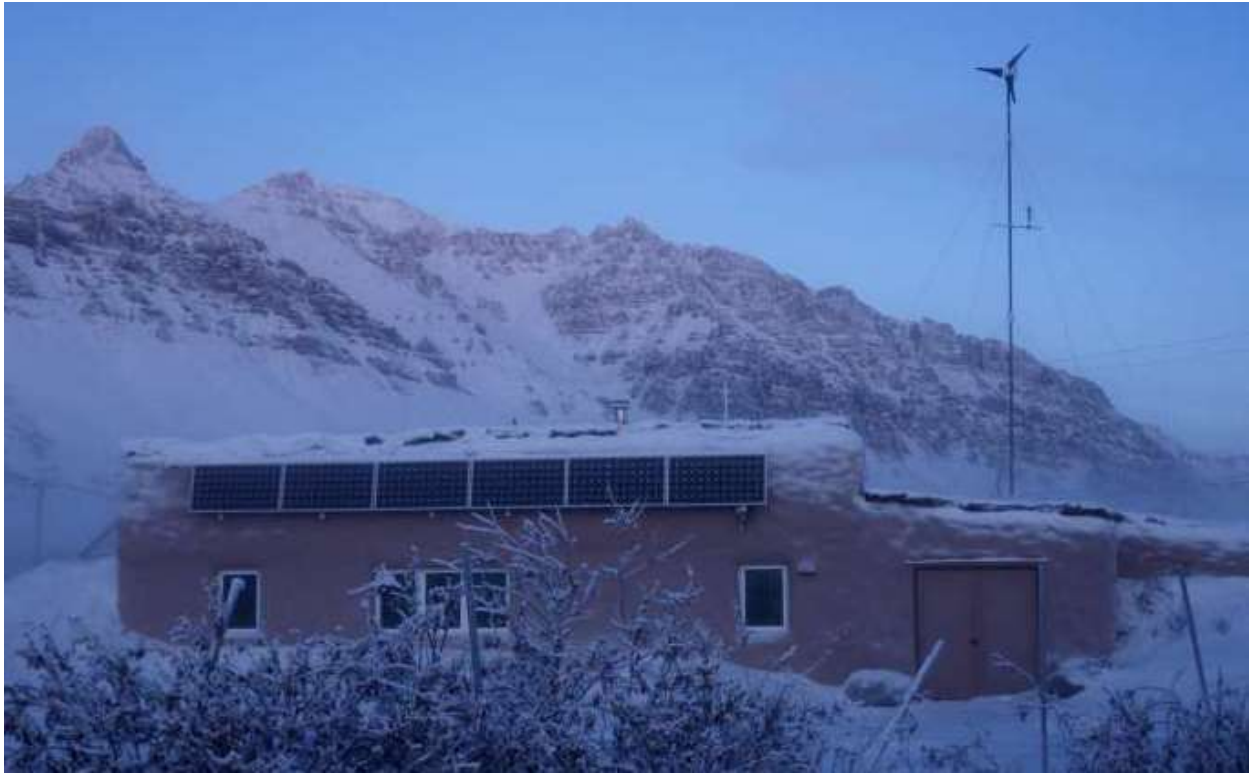
Figure 33: Winter view of the completed Anaktuvuk Pass Sustainable Northern Shelter Project (Hebert, 2010)
