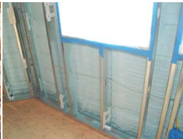
Figures 127 and 128: The roof truss tension bracket and off set wall with bracing (CCHRC 2011)
