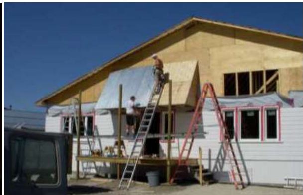
Figures 60 and 61: A double wall and solar features on the E9 House (Craig 2009)
