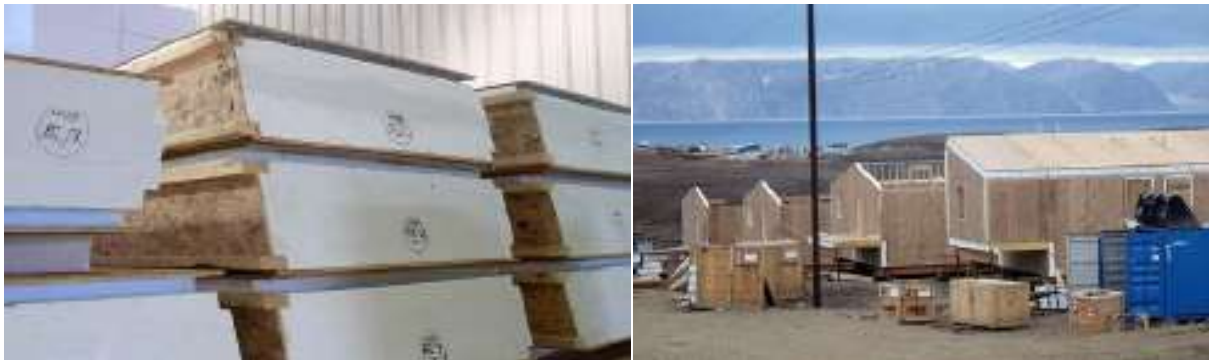
Figure 131 and 132: Tuktu panels and houses being assembled in the community of Pangnirtung (Armstrong 2010)
