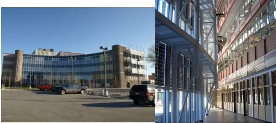
Figure 96 and 97: Canada Public Works Building, Yellowknife (Semple 2010)
