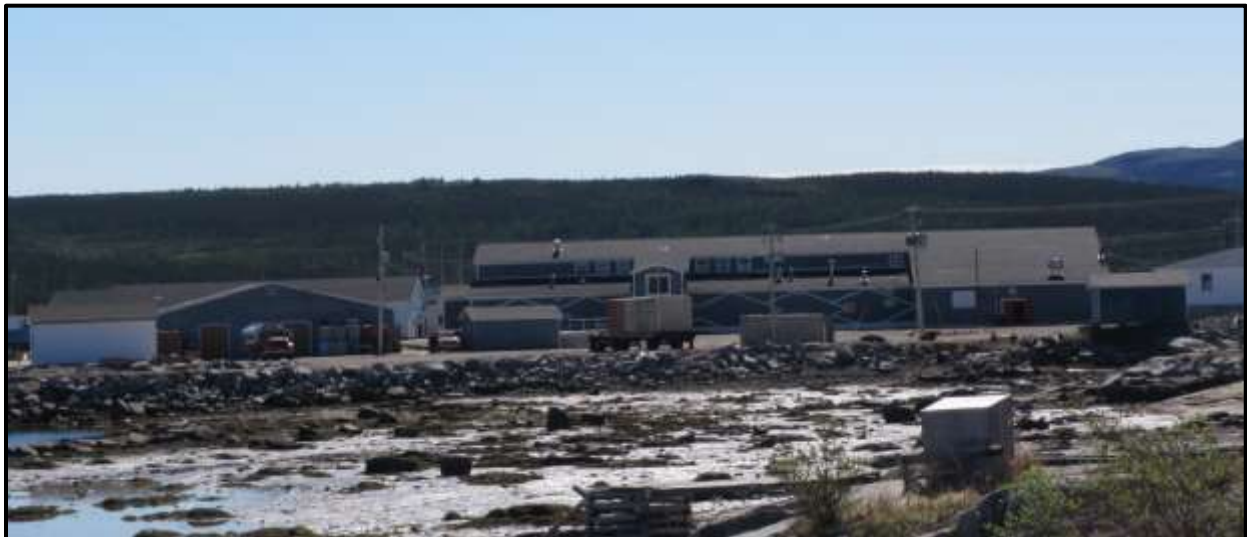
Makkovik Fish Plant
