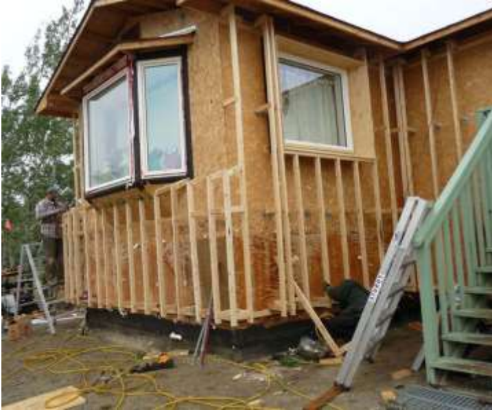
Figures 65 and 66: Installing the truss wall (Korn 2010)
