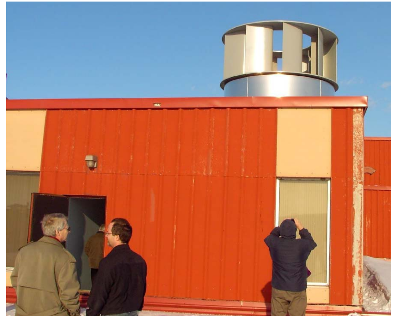
Figure 77: Windmill at Rankin Inlet, Nunavut / Vertica Vertical Wind Axis Turbine (Semple 2009)
