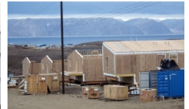
Figure 131 and 132: Tuktu panels and houses being assembled in the community of Pangnirtung (Armstrong 2010)
