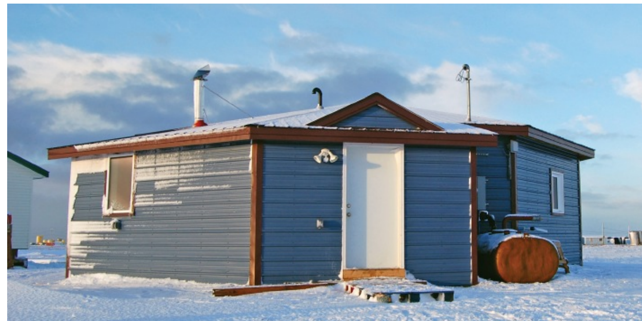
Figure 38: The Completed Quinhagak Sustainable Northern Shelter Project (CCHRC, 2011)
