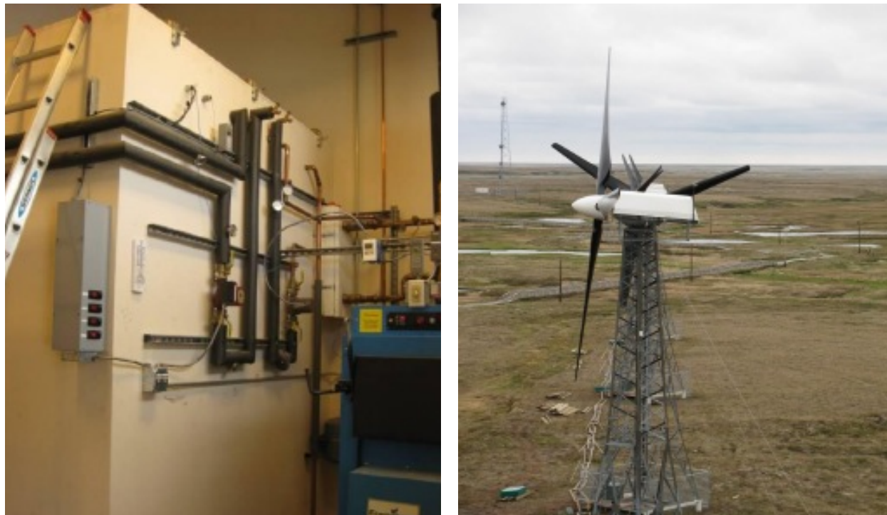
Figures 90 and 91: Thermal Storage Tank and Alaskan Windmill (Craven et al 2013)
