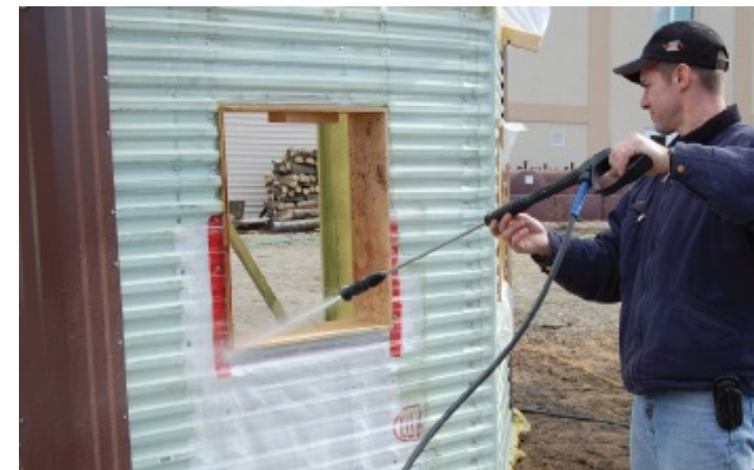
Figure 36: Wall Water Test and Assembled Wall Panels (CCHRC, 2011)
