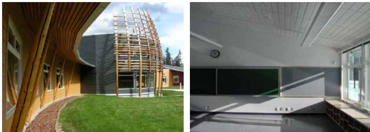
Figure 95: The importance of balancing the need for long overhangs and windows that will allow low winter light is demonstrated in the design for Tantalus School, Carmacks, Yukon by Kobayashi Zedda Architects (Zedda 2010)
