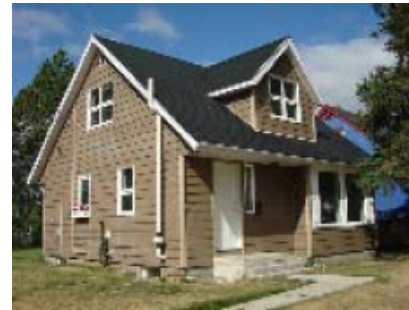
Figure 62: The House and the roof detail (Korn 2010)
