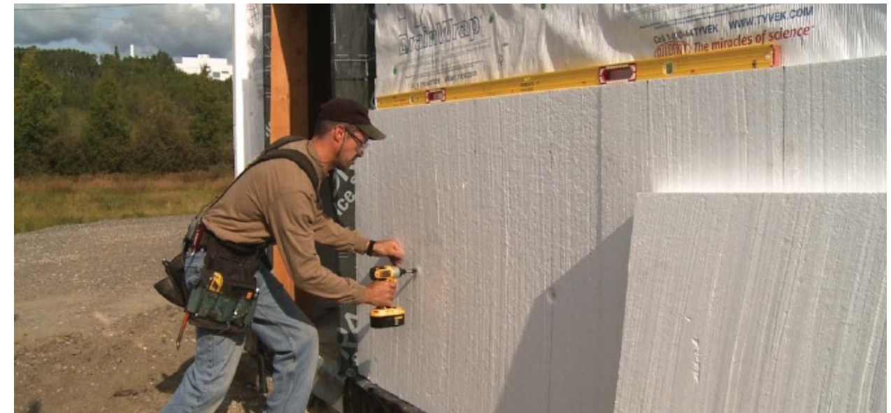
Figure 57: Installation of continuous exterior insulation as part of the REMOTE Wall (CCHRC 2009)
