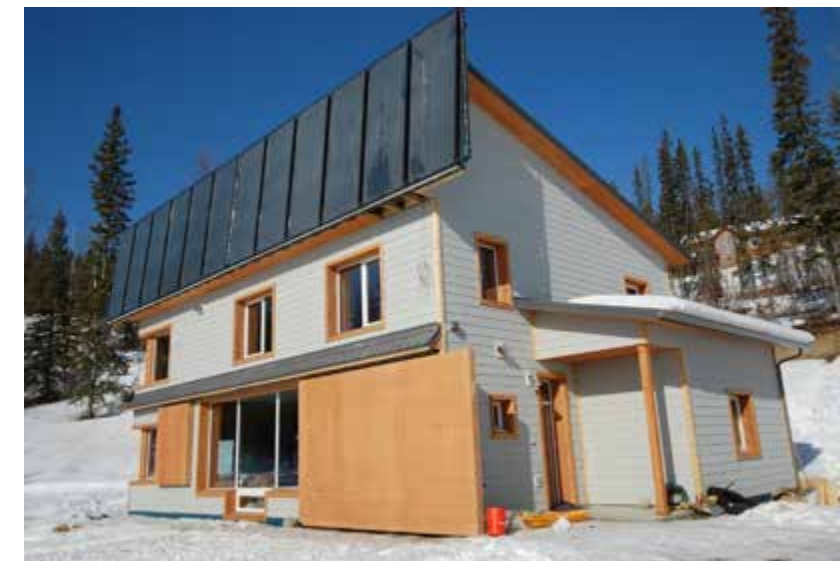
Figure 53: Passive House construction details with added solar thermal heating and exterior insulated window shutters for the severe climate of Fairbanks, Alaska (Chlupp, 2012)
