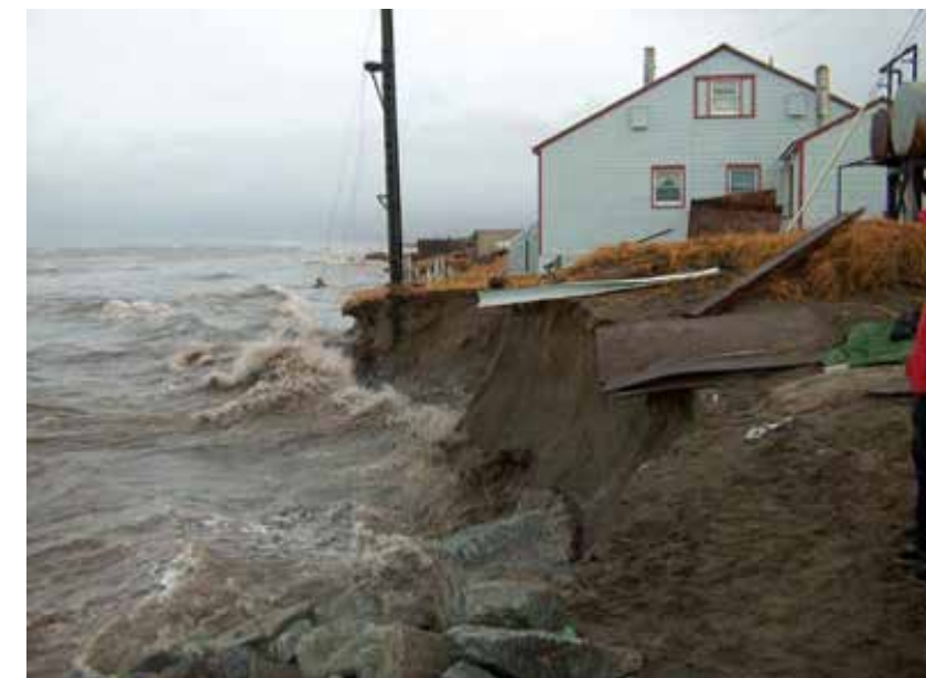
Figures 112 and 113: Impacts of Coastal Erosion in Shishmaref, Alaska (retrieved from http://multi-point-foundations.com/ )
