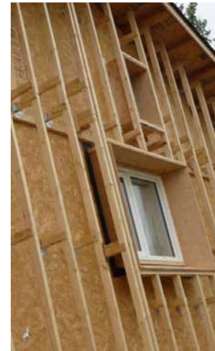
Figures 65 and 66: Installing the truss wall (Korn 2010)
