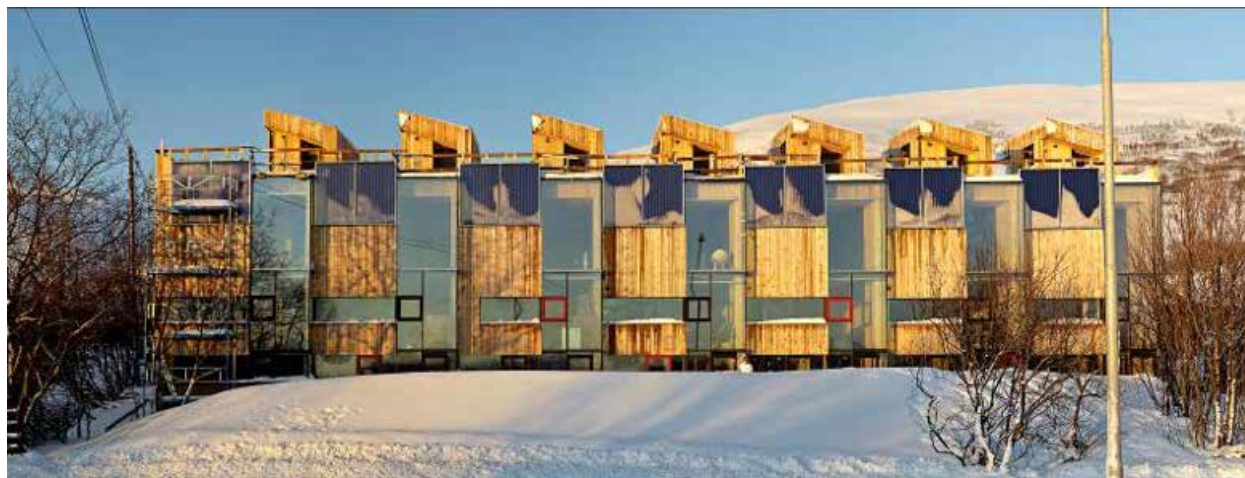
Figure 52: Multi-unit Passive House in Tromsø, Norway (Steinsvik, 2010)
