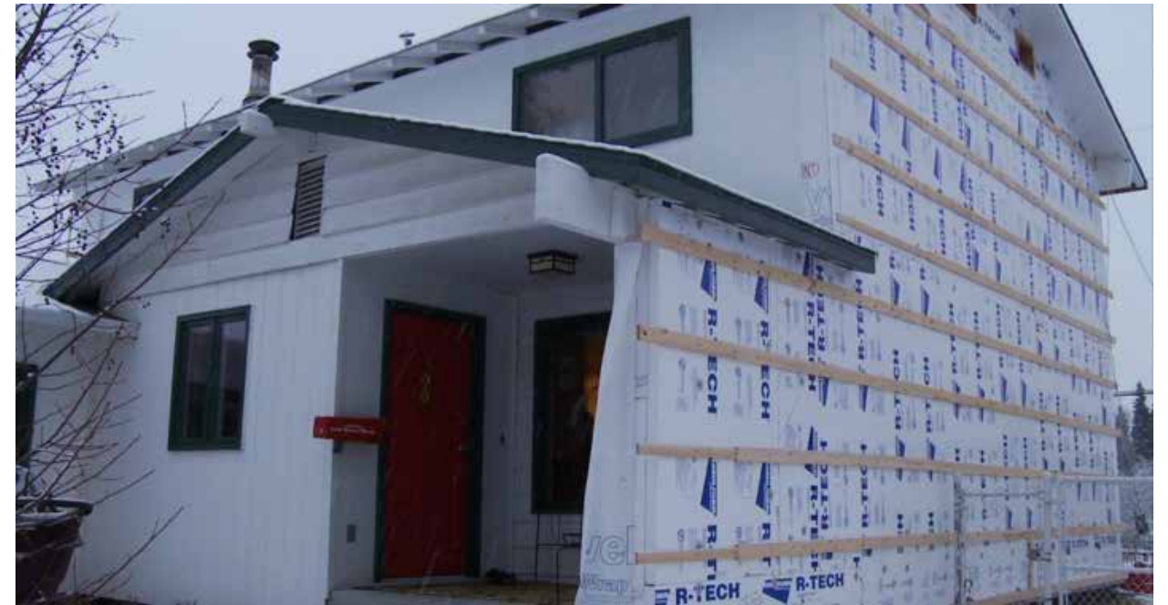
Figure 71: A REMOTE Wall Retrofit in Alaska (CCHRC 2012)
