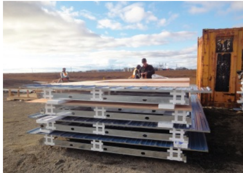
Figure 37: Wall Water Test and Assembled Wall Panels (CCHRC, 2011)
